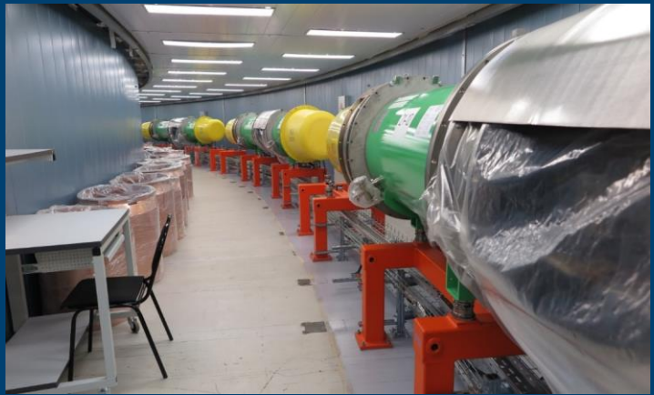
All SC magnets of the NICA Booster are manufactured, tested and installed in the tunnel inside the old Synchrotron playing the role of biological shield.
